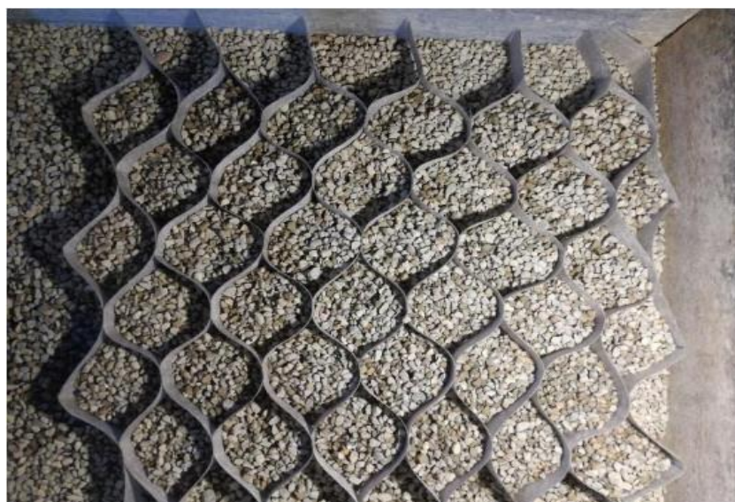
Fig. 2. A view of installed geocell in the backfill
