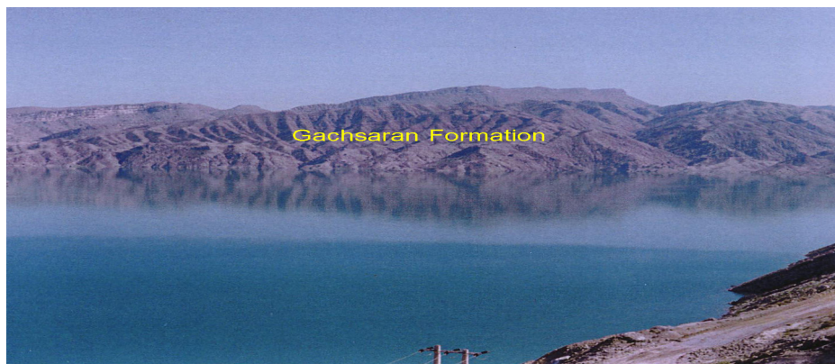
Fig. 7. The dam reservoir is covered by the very karstified Gachsaran Formation, with a number of sinkholes, caves and fissures.
