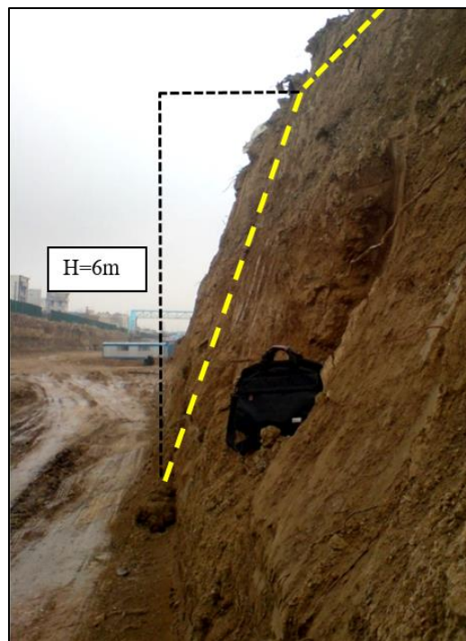
Fig. 8. The stable excavation wall with the approximate depth of 6 m and 80° in zone D 1
