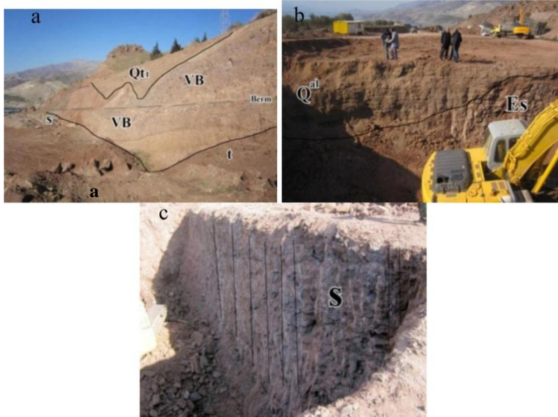
Figure 4. a) A view of the Q_t at Manjil landslide lie discontinuously on the volcanic breccias (VB) as well as VB lie unconformably tuffs (t) and sandstones (S); b) A view of the quaternary alluviums ( Q^{al} ) was deposited on the Eocene sandstones (ES). Layers of Q^{al} are horizontal; c) Layers of sandstone found in the toe slope during the cutting for the construction of bridge foundation. The figure clearly shows the high dip of the sandstone ( 65^\circ ).
